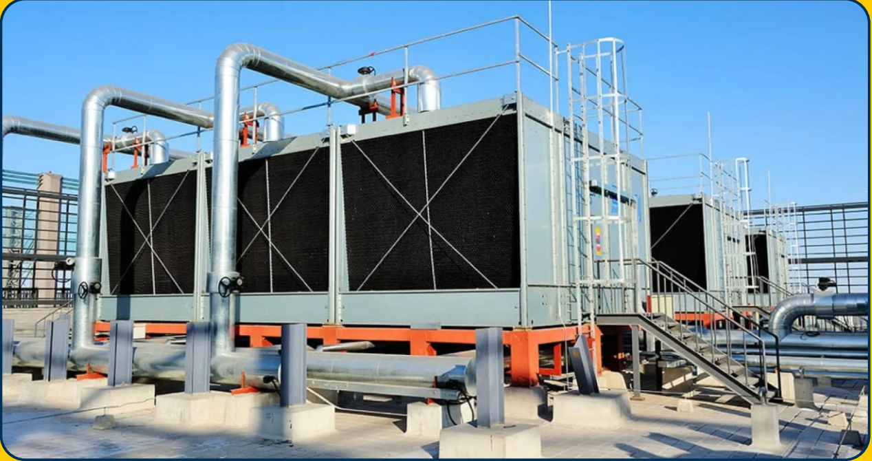
Cooling Tower and Chilled Water Pump Installation
